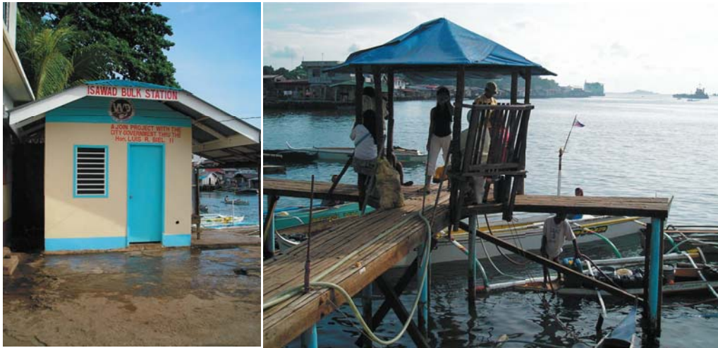
Water Kiosk operated by Isabela City Water District
